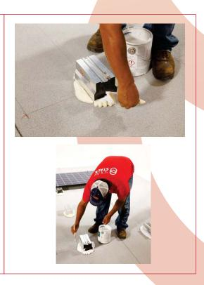
Examples with Solar Stack mounts installed on the Tile roof
