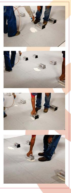
Install Solar Stack pedestal into fresh adhesive and allow to cure in accordance with adhesive manufacturer's recommendations. Solar Stack pedestal should be placed into foam within 1-2 minutes after foam is dispensed.
