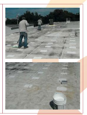
Determine the spacing of Solar Stack pedestals for your solar array design. Surface Preparation. All roof surfaces must be free of any debris, dirt, grease, oil, and standing water before adhesive is applied. Follow adhesive manufacturers application instructions.
